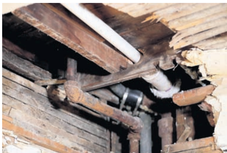
In this Nov. 8, 2018, file photo, a lead pipe, left, is seen in a hole the kitchen ceiling in the home of Desmond Odom, in Newark, N.J.
